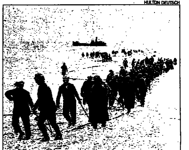
Transatlantic cable is hauled ashore at Land's End in 1926
